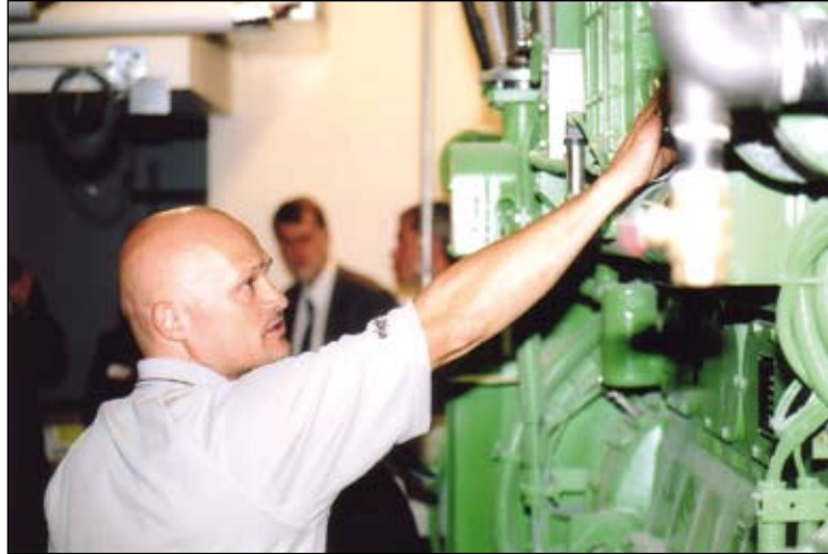
Senior Energy Engineer Vito Casola points out features of the GE Jenbacher natural gas engine-generator set at Villa Colombo Vaughan.
